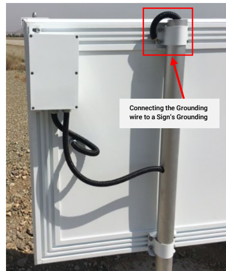
Figure 4-18 Earth Ground
