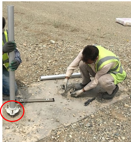
Figure 4-8 Installation (Assemble Aluminum Pipes on base plate)
