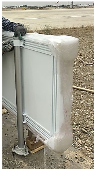
Figure 4-11 Installation (Picture C)
