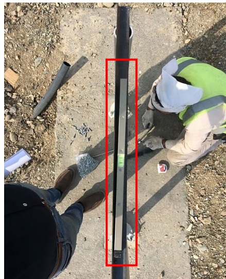
Figure 4-7 Installation (Leveling the Poles)
