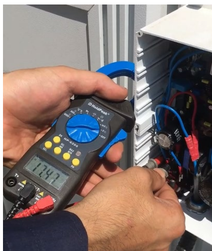
Figure 6-11 Check the output voltage and voltage across the link terminal
